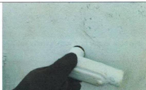
Obsolete conduit entering tank roof is loose
