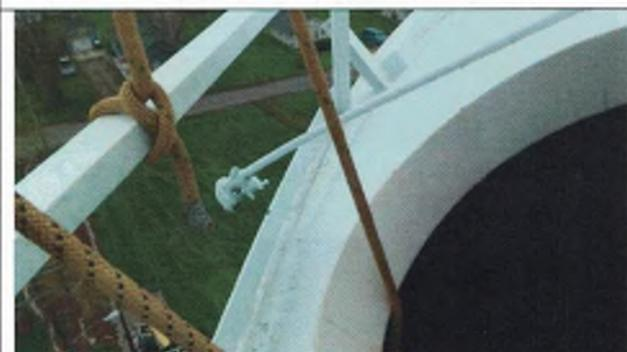
Cut off obsolete conduit on exterior roof
