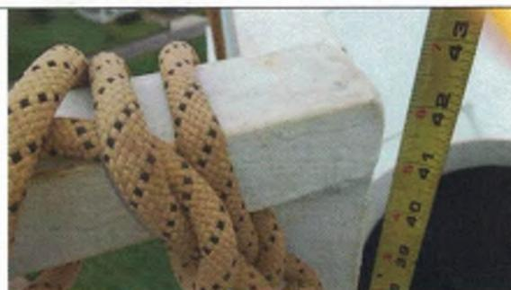
Roof handrail is 42" in height
