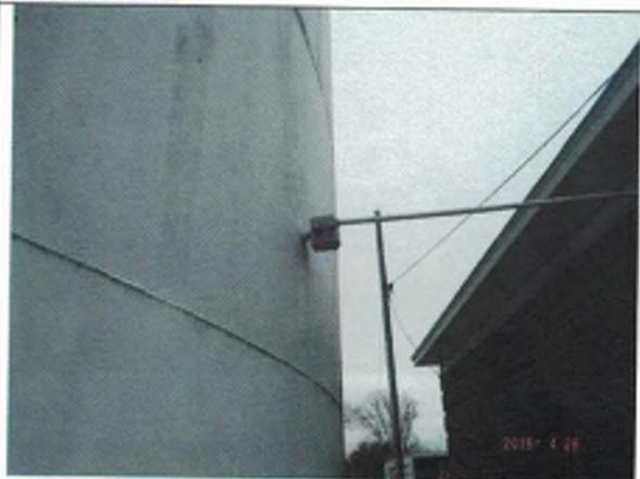
Conduit for cathodic protection entering the north sidewall
