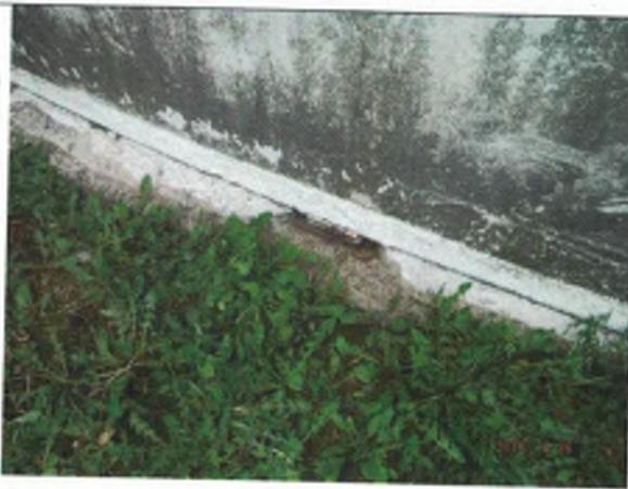
Spalling of foundation
