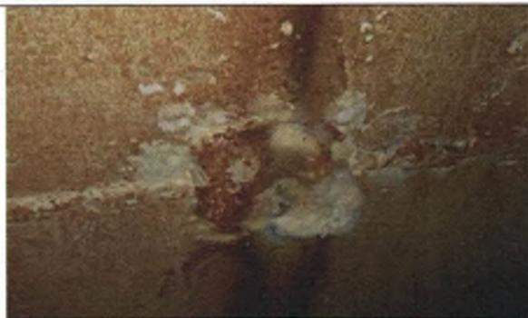
Apparent pit repair on interior sidewall seam
